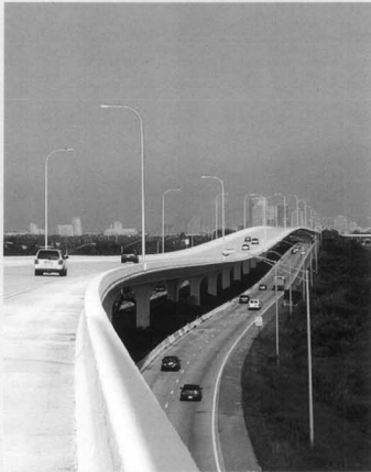
Selmon Crosstown Expressway
