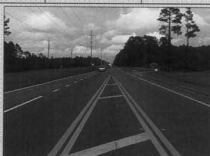
NW/NE 53 rd Ave Constructed: 2005
