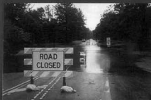
AFTER: Looking north after Hurricane Frances
