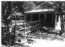
Home Repair Program: Wheelchair Ramp built
