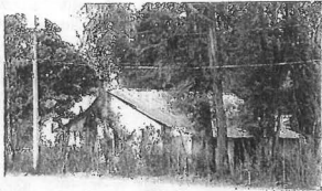
This abandoned structure faces Newberry's downtown on SR-26, which can have a detrimental effect on future commercial investment while also posing a safety risk for the community.
